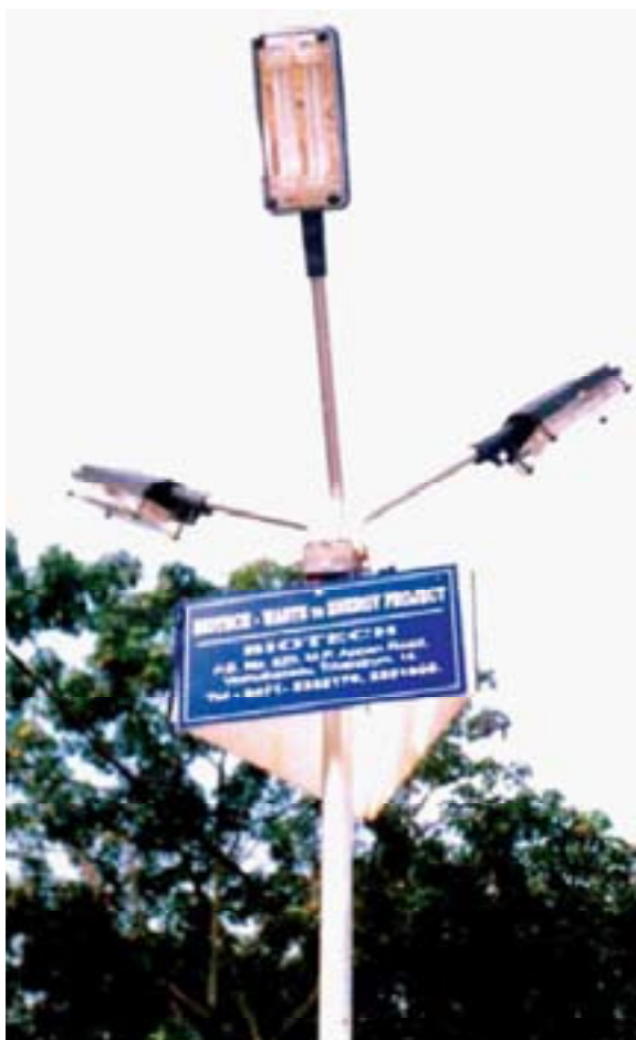
Bio-electricity lighting up streets
