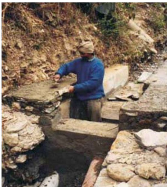
Construction of flow channel for watermill unit
