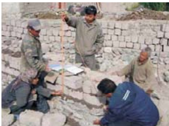
Construction of passive solar greenhouse at 14,000 feet
