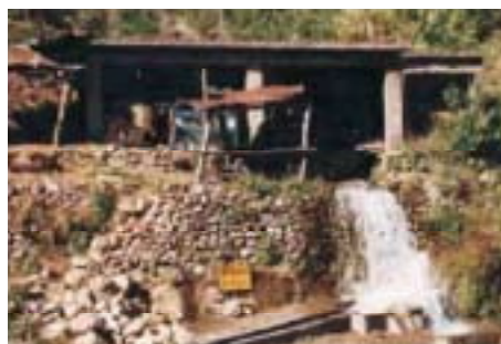
The milling house BEFORE
